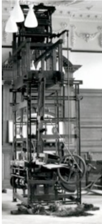
The Jacquard Ribbon Loom showing how high it is.
