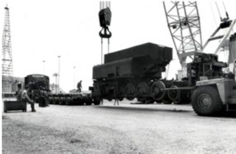
The rear unit being lifted by the crane and forklift truck.
