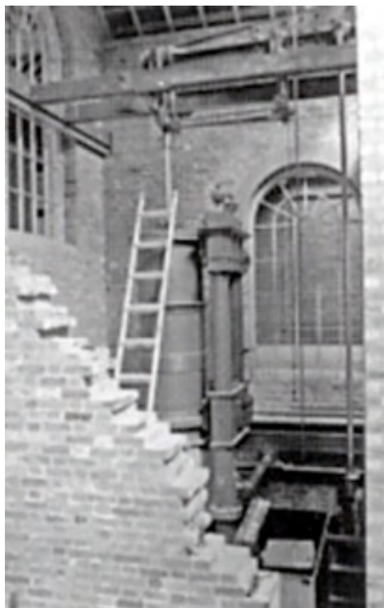
Installation of the Haydock engine at Liverpool Road showing the cylinder with parallel motion above it.
