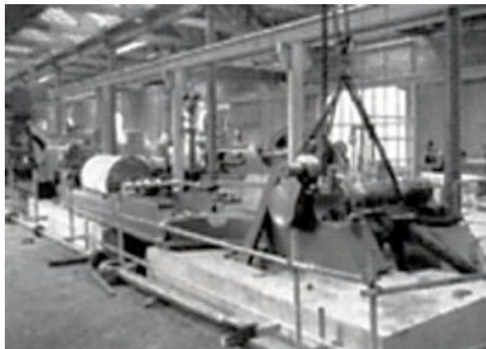
Re-erection of the Barnes Mill engine at Liverpool Road with the crankshaft being lowered on to its bearings.
