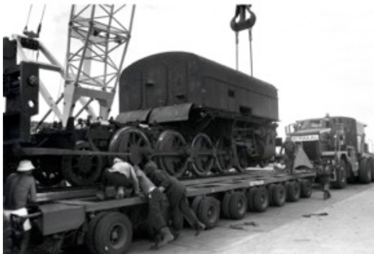
The front unit being lowered onto the trailer for towing off to the ship.
