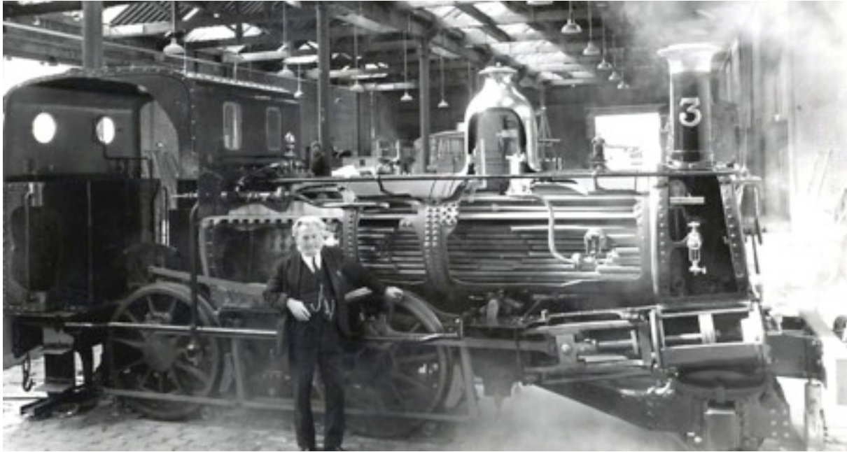
'Pender' in the Power Hall ready for display after sectioning by a Community Industry team.
